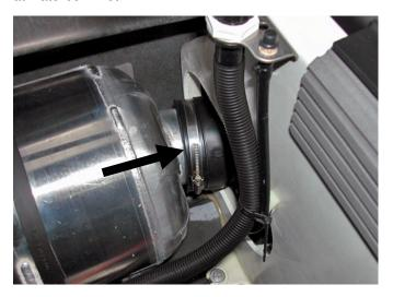
Align waterbox if necessary and secure clamp on waterbox inlet. **Note: Do not over tighten clamp.**
