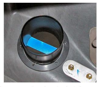
Remove excess silicone from edge of outlet flange.
